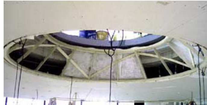
Red Bull Hangar-7 – truncated cone speaker under construction
